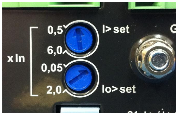
Figure 3-1 AQ110 overcurrent setting trimmers
