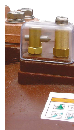
> Detail of the spark gap in a CX for protecting the primary winding.
