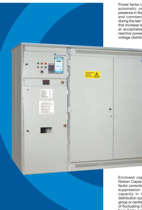
Power factor correction systems, especially automatic ones, have increased their presence in the power utilities, large industrial and commercial consumer environments during the last years. The main reason behind this increase is the need to maintain voltage at acceptable levels and to compensate reactive power to reduce losses in medium voltage distribution systems.
